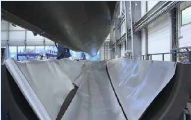
6 Insulation blankets are then placed over the infused laminate.
