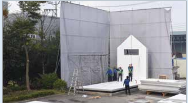
3 Panel floor was attached to the prepared concrete slab, and two panels forming one gabled end-wall were erected first, attached to each other and the floor, using a proprietary adhesive and composite profiles.
