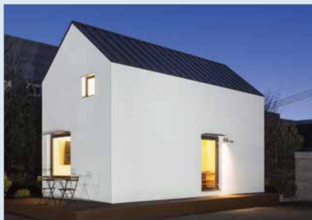
8 By day seven, the 45m 2 house was complete, including interior paint, wood flooring, exterior stucco and paint, lighting and plumbing fixtures, Google Nest IoT system, ventilation and final finishes.
