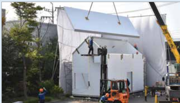
5 Two panels were then attached to form the roof.
